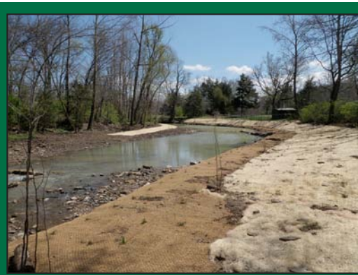
Niokaska Creek in Sweetbriar Park facing south after construction
