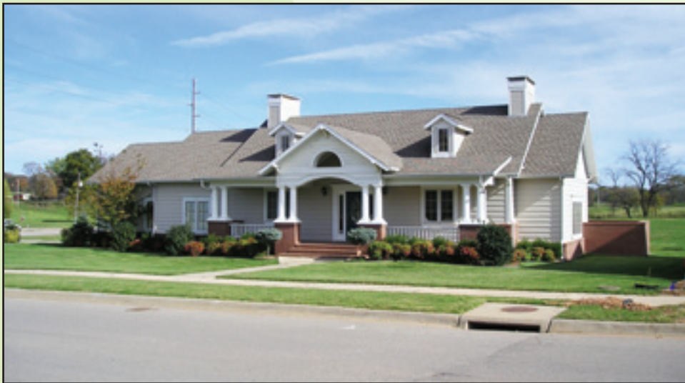
Believe it or not, that's a lift station in the Har-Ber subdivision in Springdale. Brad Hammond, president of McGoodwin Williams & Yates in Fayetteville said his firm designed the lift station so that it would blend in with the surrounding neighborhood and not adversely impact property values.
