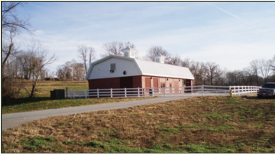
This lift station, designed to fit an agricultural area in Washington County, netted McGoodwin Williams & Yates in Fayetteville the Engineering Excellence Honor Award from American Council of Engineering Companies of Arkansas.
