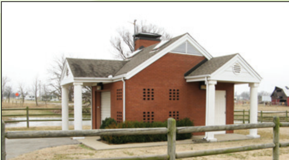
Brad Hammond, president of McGoodwin Williams & Yates in Fayetteville, said designing lift stations to blend in with surrounding areas can make projects enjoyable for designers.
